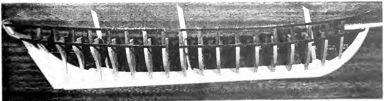
HAWK'S NEST, OR CROW'S NEST, HALF-MODEL, WITH KEEL AND DEADWOOD FORM SHOWN. Mould-sections were at alternate frames, and sheer and deck lines were indicated by the use of battens tacked to moulds. The keel detail shown is unusual. One of the older forms of builder's half-models, this one, in the author's collection, is of the 3-masted Baltimore schooner Flying Fish of about 1806. (Smithsonian photo 45607-c.)
